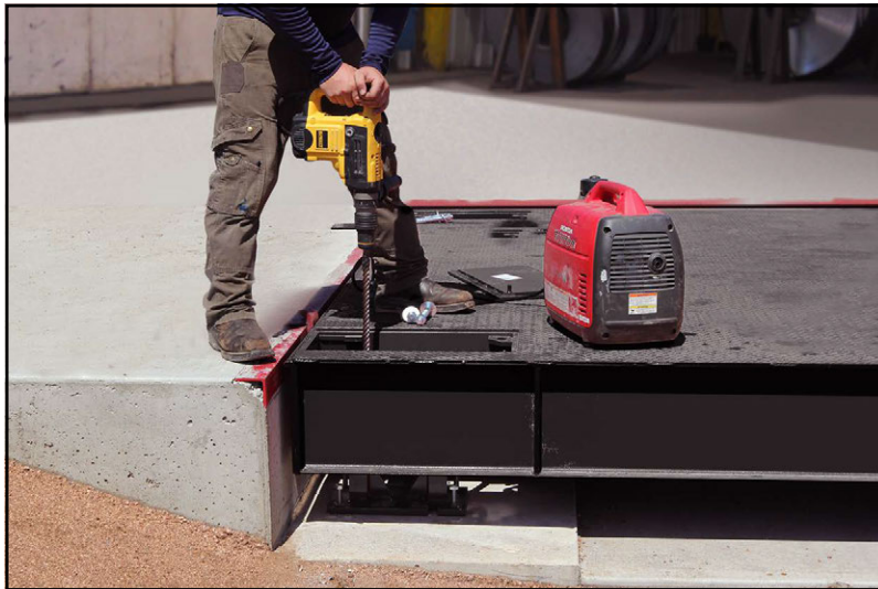
Figure 3-14. Drill Anchor Bolt Holes
